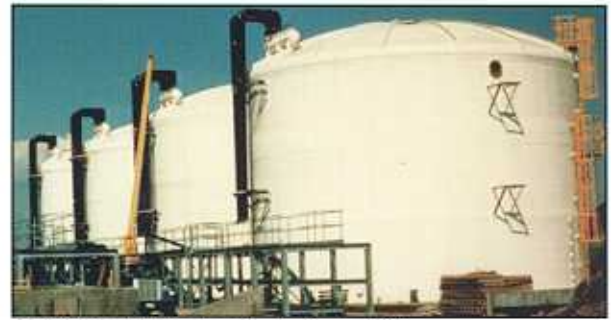
48' X 32' Waste Water Neutralization Tanks, 1988
