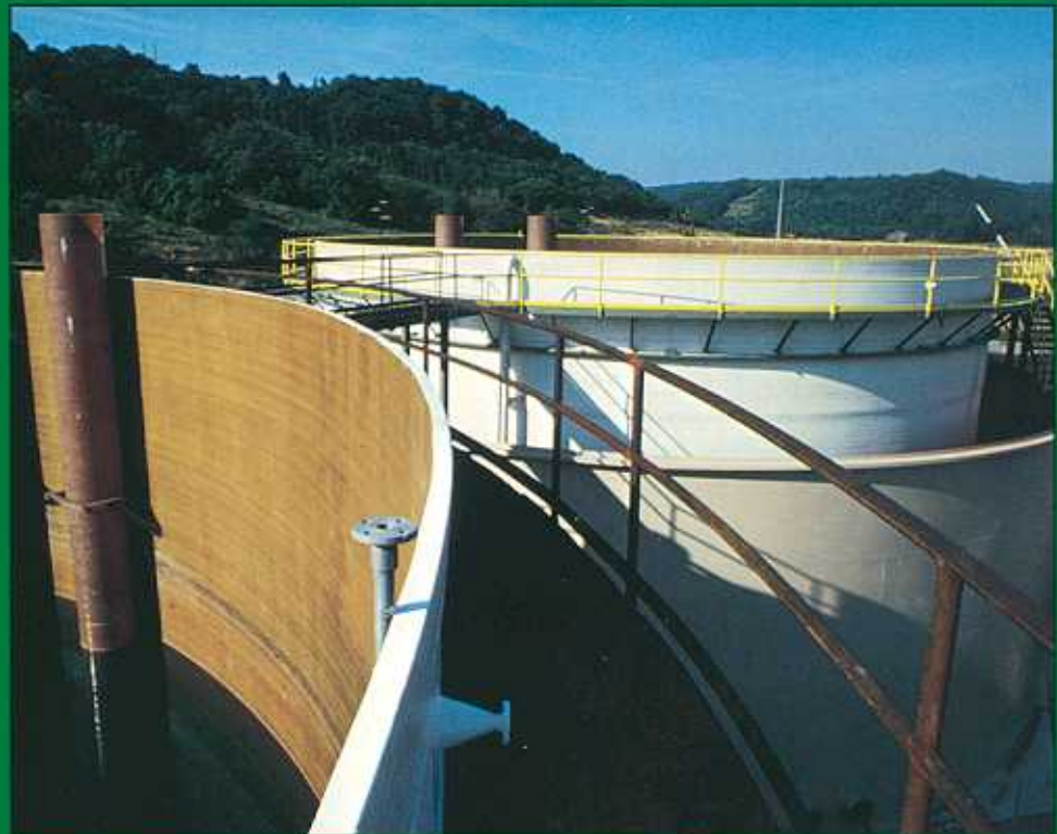
Waste Water Tanks, 65' Dia x 40', 1993
