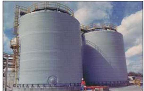
40' X 37' Chlorine Dioxide Storage Tanks, 1989
