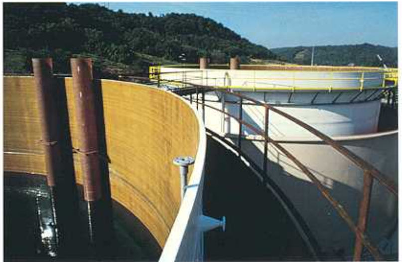
65 ft. dia. neutralization tanks
